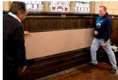
23 Radiators like the one above will be removed. They will all replaced with modern heating cooling units like the one being held in place for a trial fit. When these are painted and finished they will all but disappear and we will have the heat and cooling we need.
